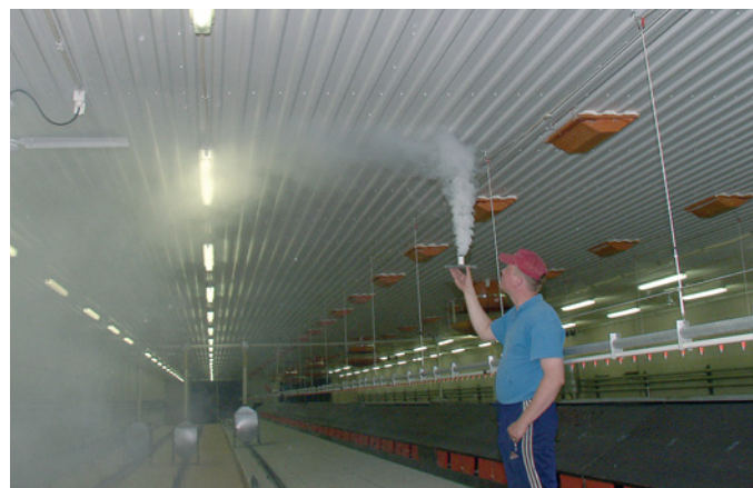
Smoke is used to visualize the air circulation inside an animal shelter in order to optimize the design of the ventilation system.
